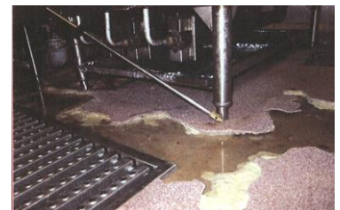
Thin Film Topping shows damage through to the substrate resulting in early failure or premature wear
