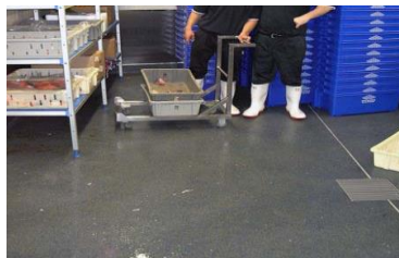
Heavy Duty Floor Topping has surface chipping but is structurally sound
