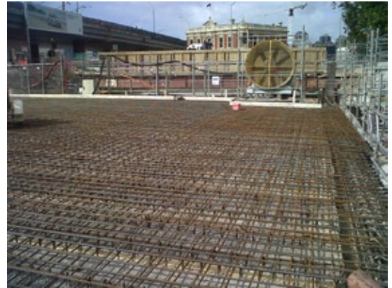
Preparing a heavy duty concrete slab
