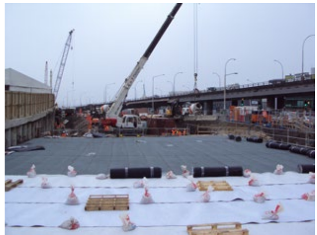
Membrane onto a concrete slab
