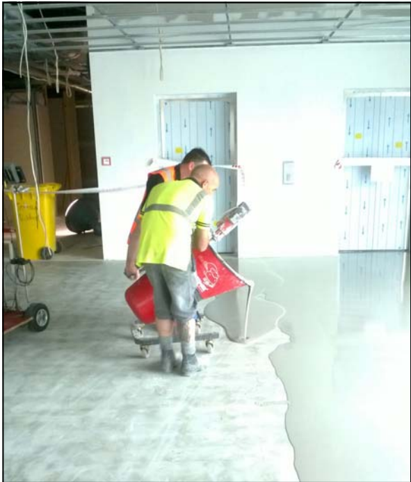
Applying P510, a self smoothing compound
