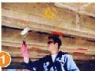
1 Apply MBrace Primer onto prepared concrete substrate
