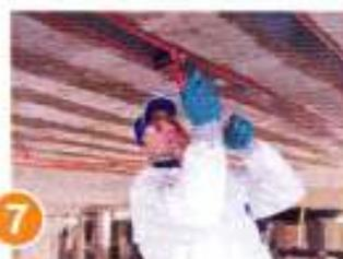
7 Roll MBrace Laminate to secure onto substrate and clean up excess
