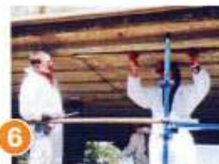
6 Position MBrace Laminate and apply to substrate
