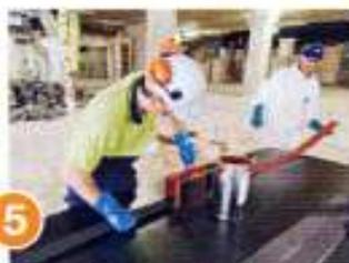
5 Apply MBrace Laminate Adhesive to Laminate
