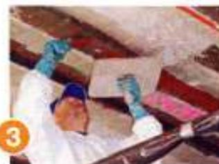
3 Apply MBrace Laminate Adhesive to substrate
